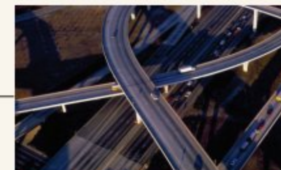
On going 6 Lane Highway near Walajahbad for faster connectivity
